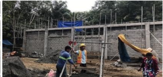
(On-site construction of the Rubber Cup Lump Consolidation Warehouse)
