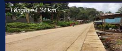
CONTRACT PACKAGE 3-C Project Cost: ₱157.76 Million
