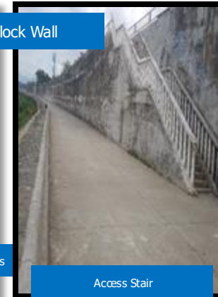
Wet Stone Masonry and Handrails
