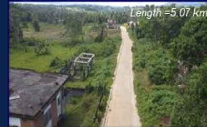
CONTRACT PACKAGE 3-A Project Cost: ₱234.41 Million
