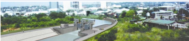
Pasig-Marikina River Channel Improvement Project, Phase IV
